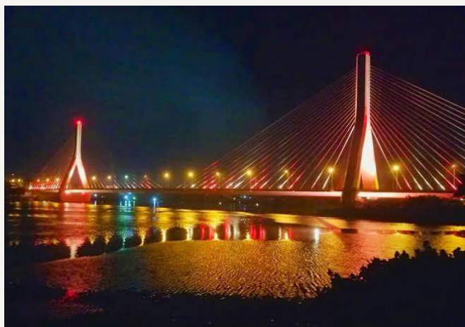
Uganda Jinja Bridge
